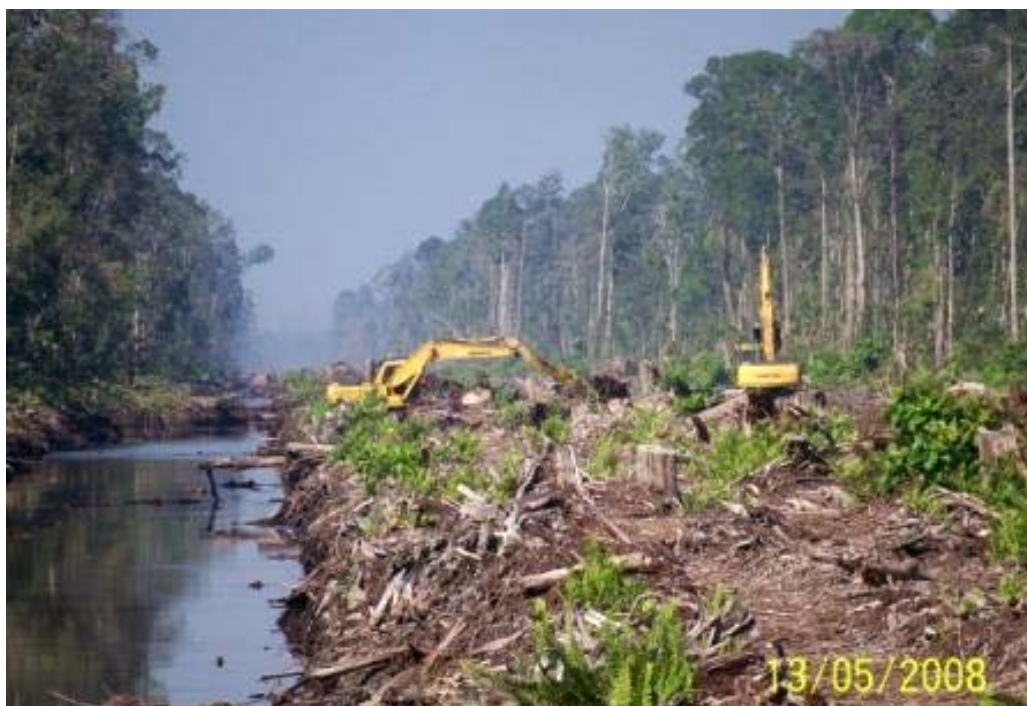
Image 1. New logging road construction by APP and its affiliated company in peat swamp forest of Senepis (N. 1 57 12 E, 101 13 15). It involves the clearing of a 50-meter swath of little-disturbed natural forest -- 25 meters width for the road and 12.5 meters width on both sides for drainage canals.
